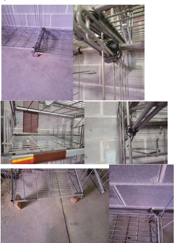
As you can see the old lockers were being held together with zip ties, ropes and various other straps to keep them from falling apart. They were also starting to pull away from the anchors that were attaching them to the walls. These lockers had far out lasted their usability within the Fire department.
